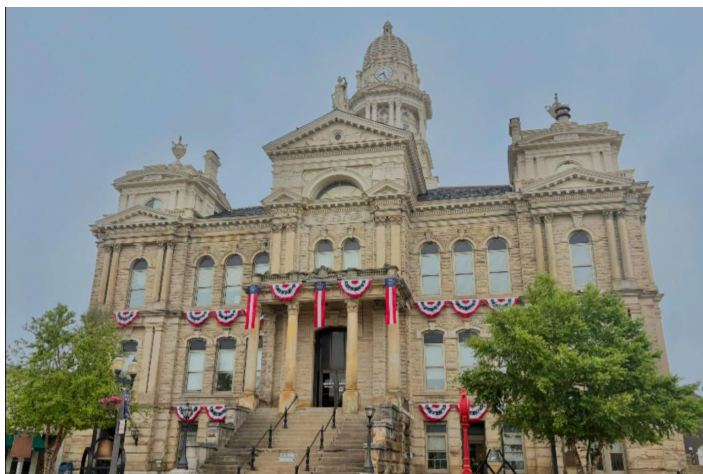
The Belmont County Courthouse.
