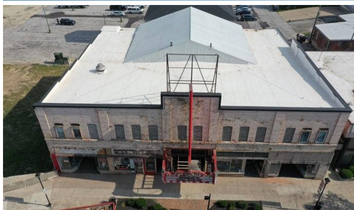
The St. Marys Theater and Grand Opera House exterior during renovations.
