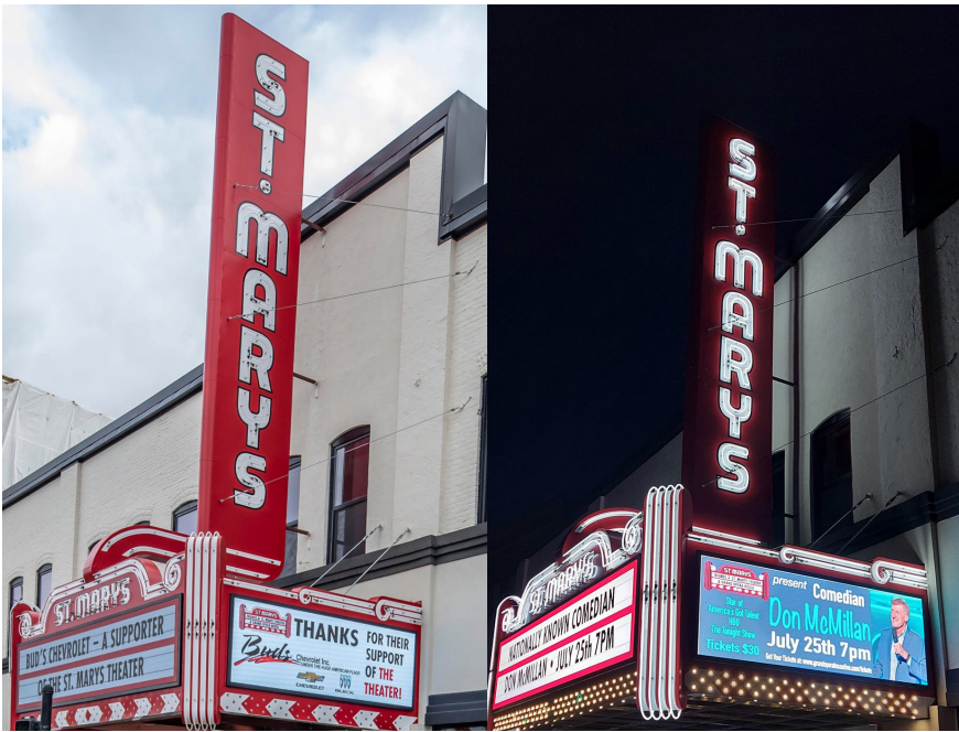
The newly-restored marquee, with the original letter board replaced by a new digital board to allow for the display of multiple and more complex visuals.
