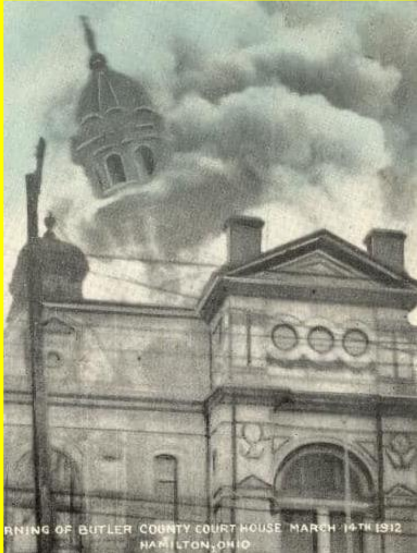
Butler County Courthouse Fire 1912
