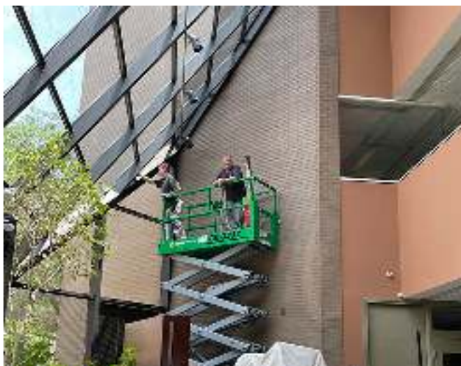
The tinting of the atrium window.
