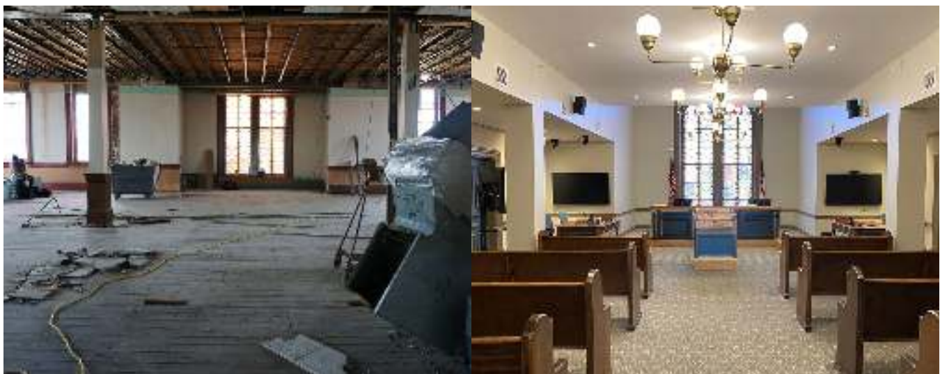
Delaware County Courthouse Hearing Room, before and after
