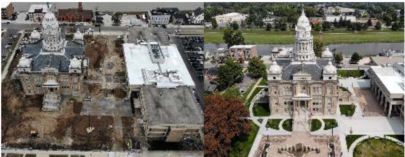
Miami County Courthouse, during and after renovation
